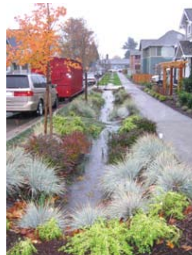
Bioswales retain and treat stormwater in High Point
