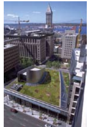
Green roof atop Seattle's City Hall
