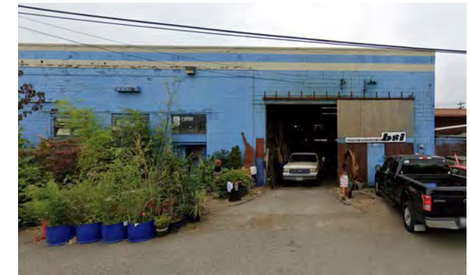
Equinox metal fabrication shop
