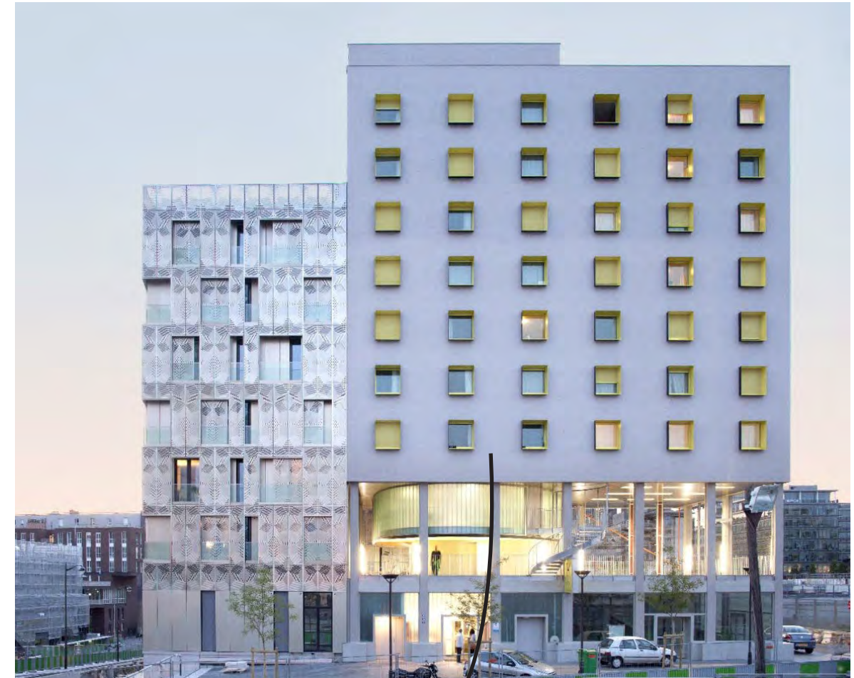
Housing massed as simple volume above concrete plinth with commercial + communal spaces
