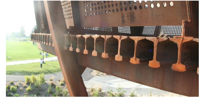
Reclaimed railroad rails, or other reclaimed materials, can become deck paving at the corner eddies.
