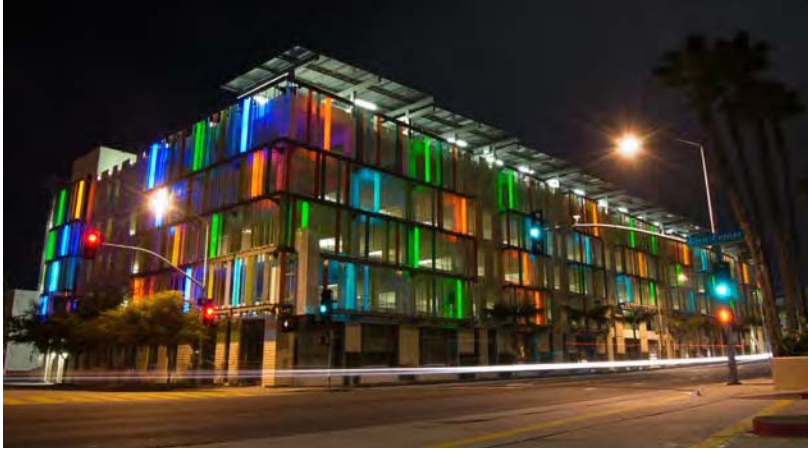
The Civic Center parking structure in Santa Monica, California, the first LEED-certified building of its type, is an excellent example of a sustainable parking option.
